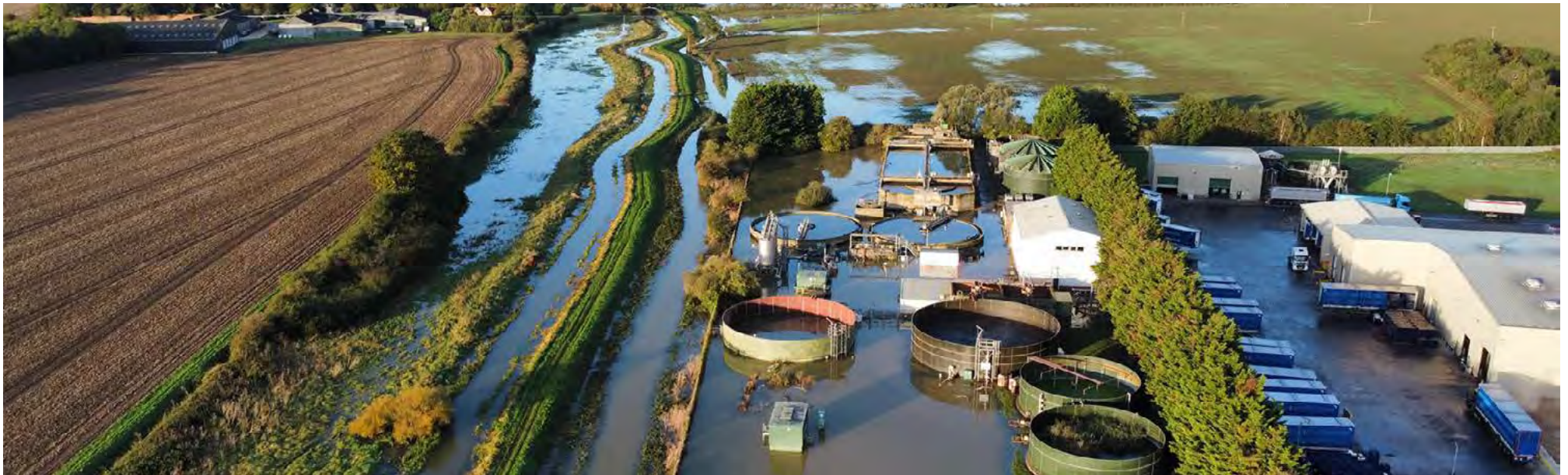
Anwick Water Recycling Centre under water.
