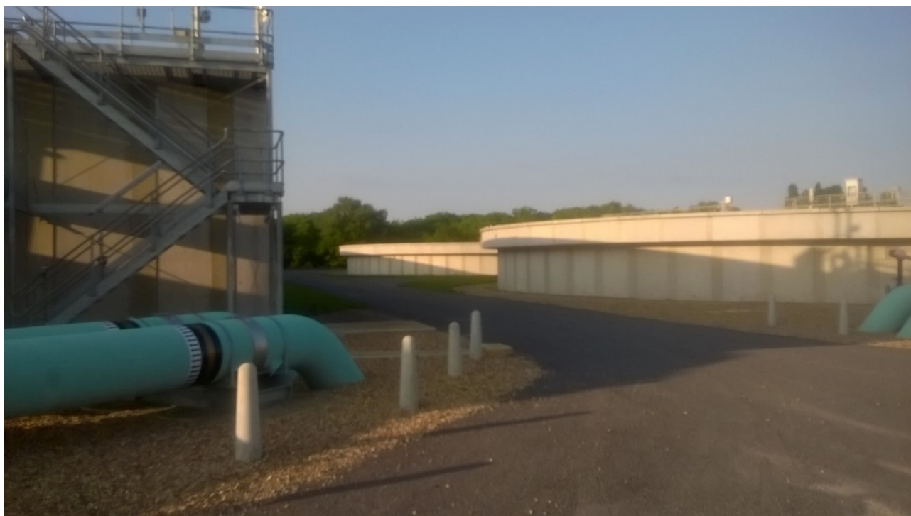
Figure 8 Example of modular precast concrete tanks
